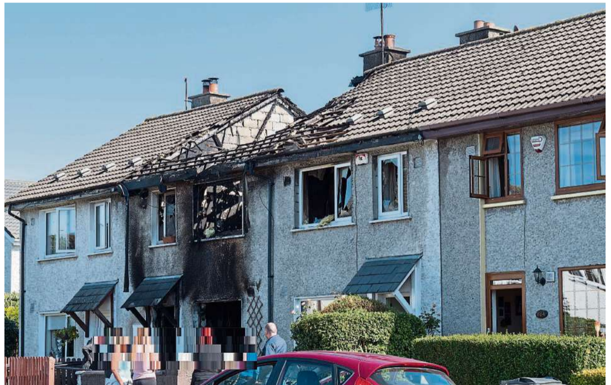
The large blaze caused extensive damage to the property's roof and upper floor. PICTURE: TONY KEANE
