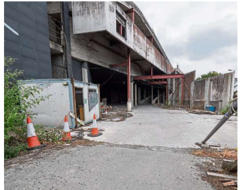
The derelict Naas Shopping Centre site. PICTURE: TONY KEANE
