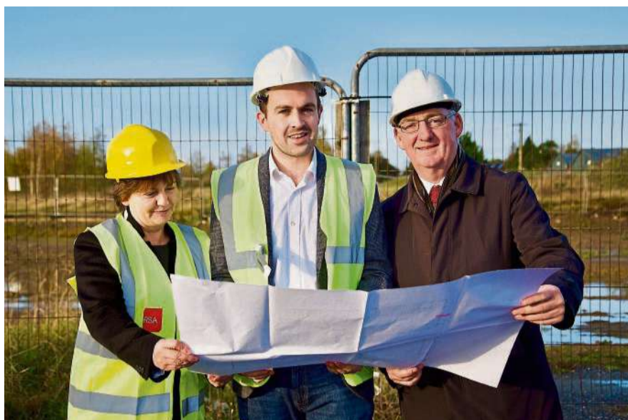
Ena Coleman, Regional Development Executive Dublin Mid East at Enterprise Ireland with Cllr Rob Power and Peter Carey Chief Executive, Kildare County Council on site as construction commences on the new MERITS Tech Hub for Naas/Kildare
