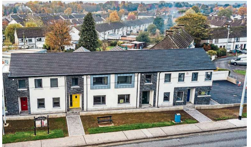
The four newly-built homes at Railway House in Naas
