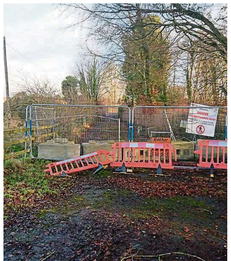
The L6042 was shut by the Council in August 2016 after a section of it became unstable due to subsidence. PICTURE: DEREK CLIFFORD
