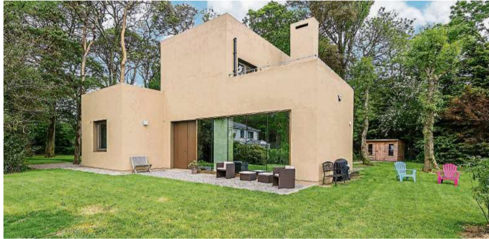
Aisling House, Bishops court, in Straffan
