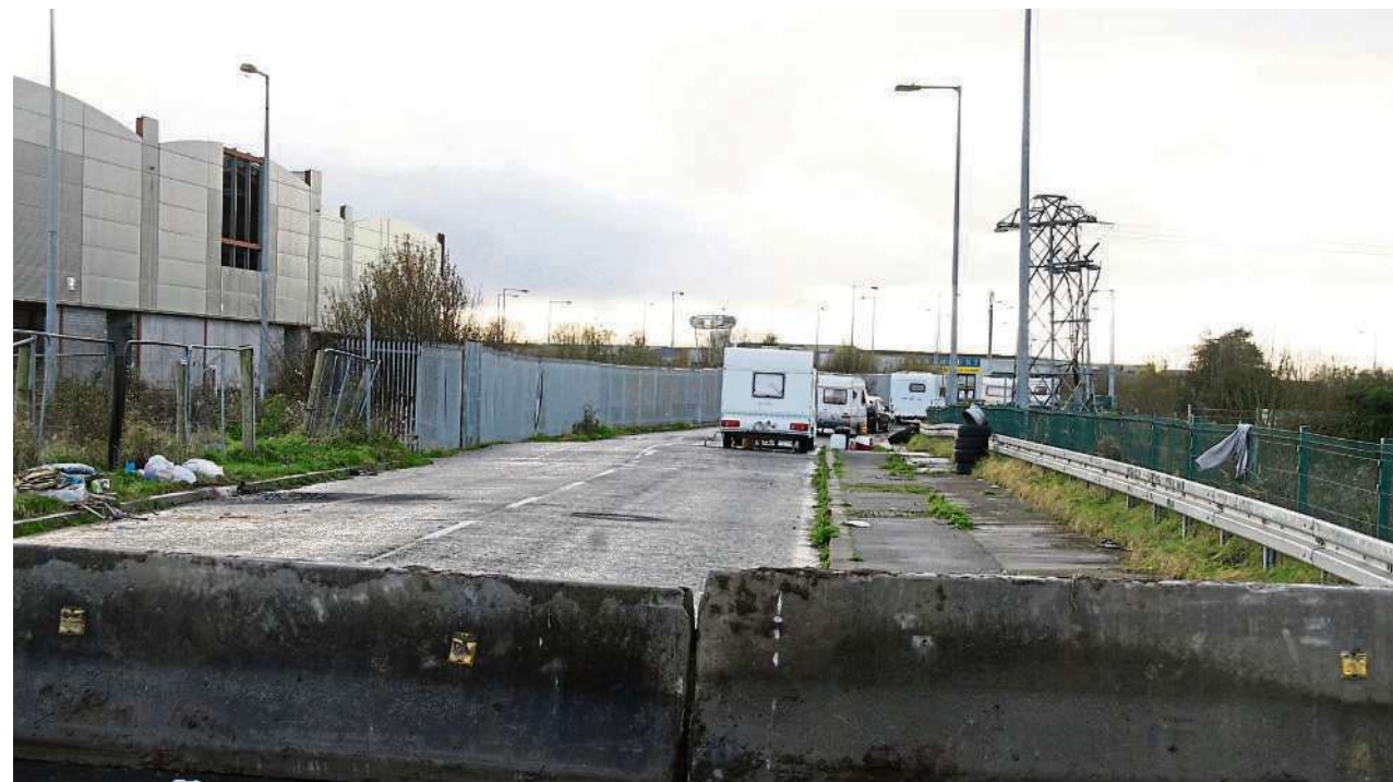
Some of the caravans which were parked near the site of the Northern Distributor Road last week PICTURE: ADRIAN BUTLER
