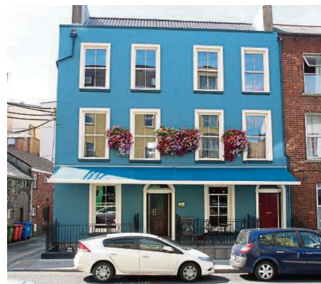
The newly-renovated Commercial Bar on Catherine Street
