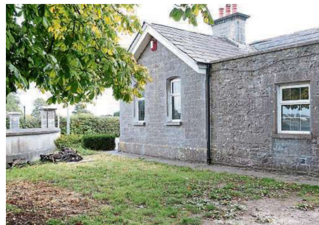
The 150-year-old protected structure sustained exterior fire damage on Friday night
