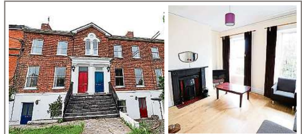
O'CONNELL AVENUE, LIMERICK 2 & 2A OLD WELLINGTON TERRACE
