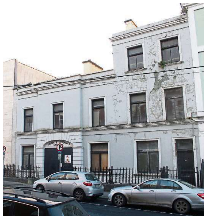
The former OPW building at Cecil Street, which is to become a 'Digital Collaboration Centre' PICTURE: ADRIAN BUTLER
