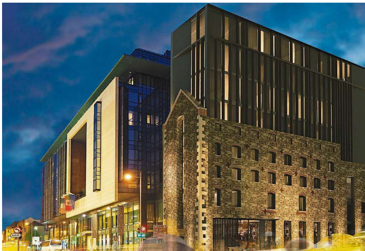
An impression of the Savoy Hotel's expansion, which has been given the go-ahead
