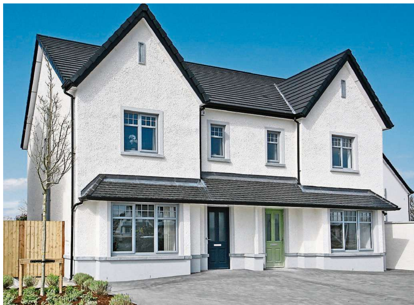
Mungret Gate: the first phase is made up of three and four bed semi detached homes
