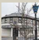
Mayorstone garda station
