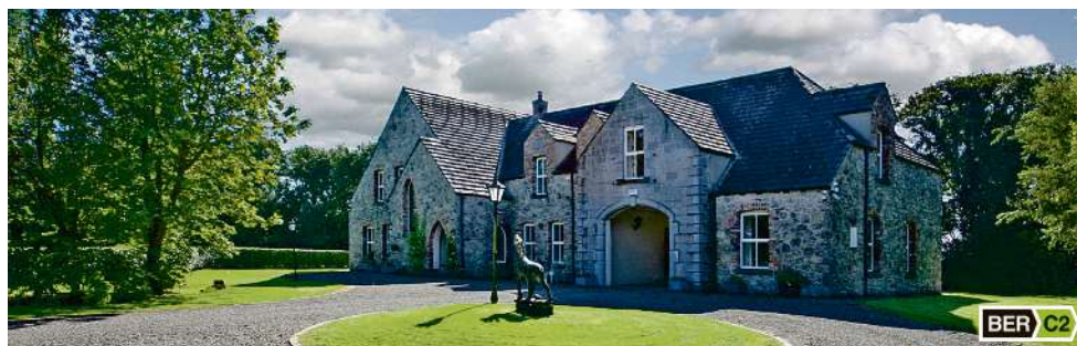
ROCKBARTON HOUSE, LEMONFIELD, CRECORA, CO LIMERICK
