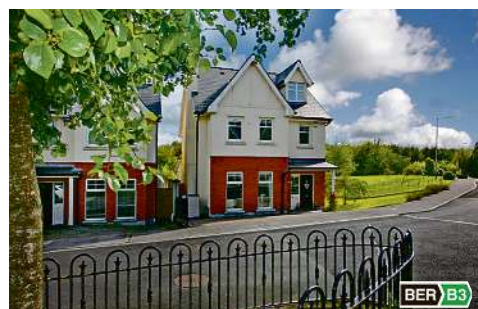
50 CAIRNSFORT, GOLF LINKS ROAD, CASTLETROY
