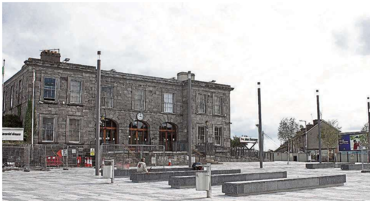
The site, which extends to 50 hectares is located behind Limerick's Colbert train station
